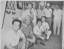
"Toal" boiler startup men in foreground: J. V. Croes, HDS Coordinator; V. P. Lacie, operator; M. Kelly, controlman; and S. Kloda, ERE. Standing: Mr. Menoal, Toal Commissioning Enginaar; N. Westler, operator; J. Park, HDS Coordinator; W. Prime, shift foreman and J. Gibbs, controlman.
